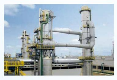
24 MW steam jet chilling plant Petro China/Sichuan refinery, cooling of 2 300 m³/h from 29 °C to 20 °C
