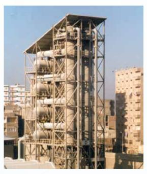
28 MW steam jet chilling plant in Egypt, cooling of 1 600 m $^{\!3}/\!n$  from 35  $^{\circ}C$  to 20  $^{\circ}C$
