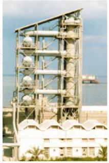
Bridge design with separate steel construction, option of a 2-tower design, 4-stage, cocurrent plant
