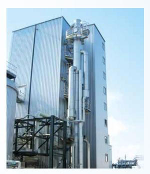
About 1.4 MW steam jet chilling plant in Stendal, cooling of about 72 m $^3$ /h from 25  $^{\circ}$ C to 8  $^{\circ}$ C
