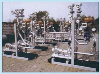
Electrically heated inplan Thermal Oil Boiler, 700 kW, 380 volts, 50 cycles, with 7 heating cartridges 100 kW each, circulating pump, control cabinet, max. outward flow temperature 300 °C.
