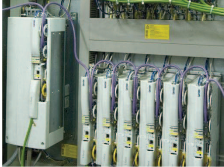
cabinet design & construction
